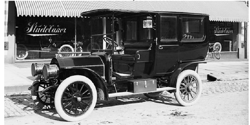
1908 Studebaker Limousine with open drivers' compartment for the chauffeur and a closed cabin for passengers
