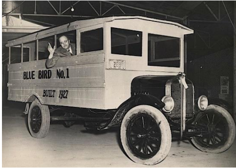
Blue Bird No. 1 the first bus constructed by A.L. Luce founder of the Blue Bird Body Co. It is based on a 1927 Model T chassis.
